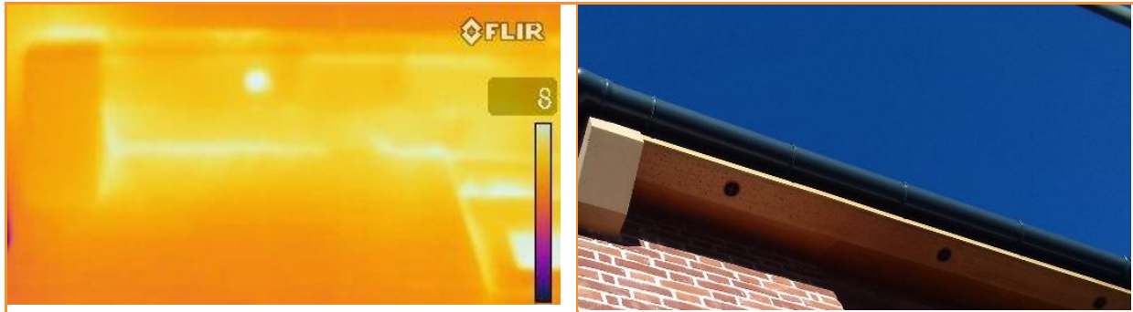
9.41: Thermographic image while building pressurised, through eaves vent & top of column
