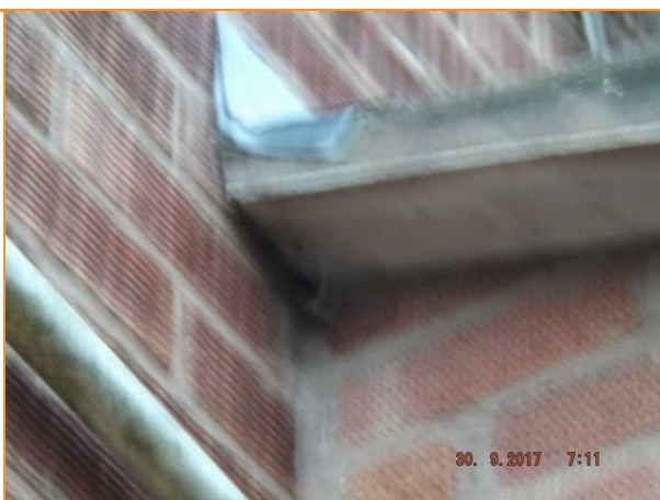
9.14: Leakage along interface between top of wall and underside of roof to lean-to extension
